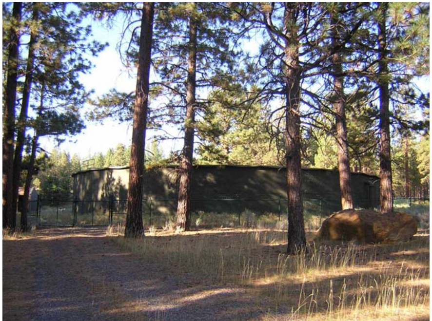
City of Sisters 1.6 MG Prestressed Concrete Reservoir
