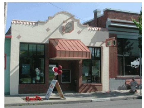
OFCCU Ridgefield building after remodel
