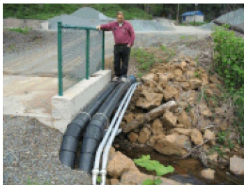
Peterson Creek bridge crossing
