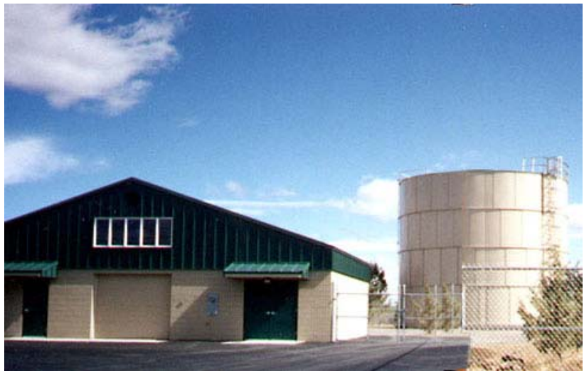
Terrebonne Control Building and Reservoir
