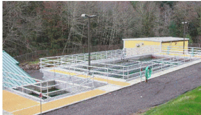
Water treatment plant site overview
