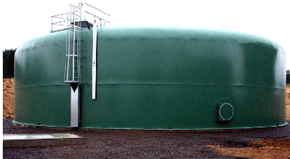
Welded steel reservoir
