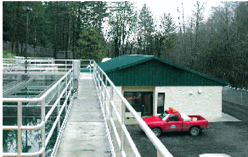
New water treatment plant building and sedimentation basin
